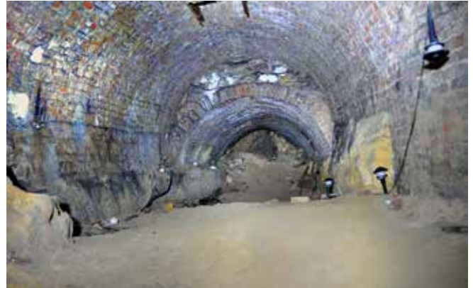
The backfilled tunnel leading to the old seafront entrance
